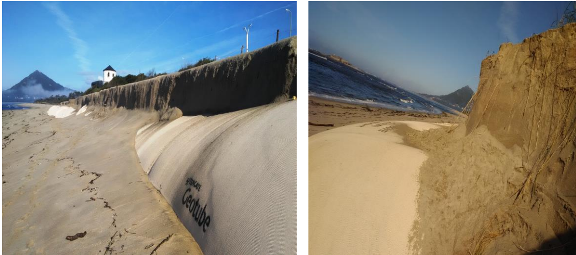
Figure 8 - Moledo beach dune after a storm in December 2019, with exposed geotube in a destroyed dune.
